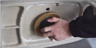
9. Turn over the toilet bowl and install the flange ring as below picture
