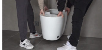
11. Move the toilet to the location where it will be installed
