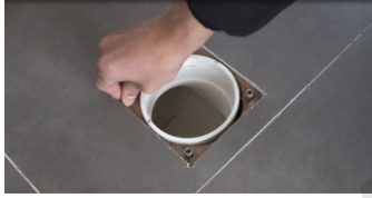
4. Put the screws into the holes
