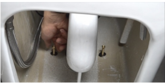
12. Make sure two holes in the bottom of the toilet align with the two long screws in the flange ring, then install it
