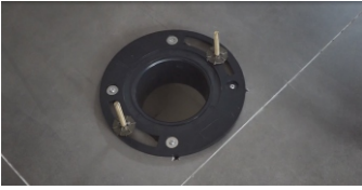
6. Install two long screws as below picture
