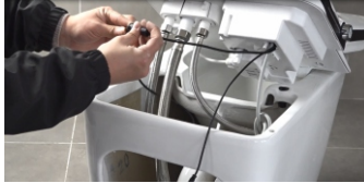
13. Put the toilet seat in the toilet and reconnecting the flexible tube and black wire
